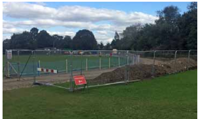
The bypass bridge (top) and flood defences under construction (bottom) © Mike Jackson
