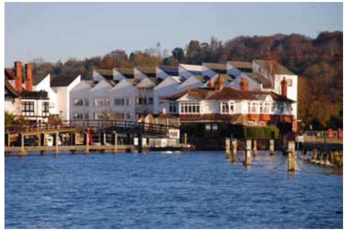
Modern housing development on the site of Marlow Mills © Mike Jackson
