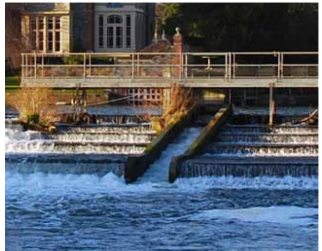
Fish ladder integrated into Marlow weir © Mike Jackson
