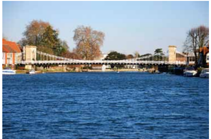
Marlow Bridge © Mike Jackson
